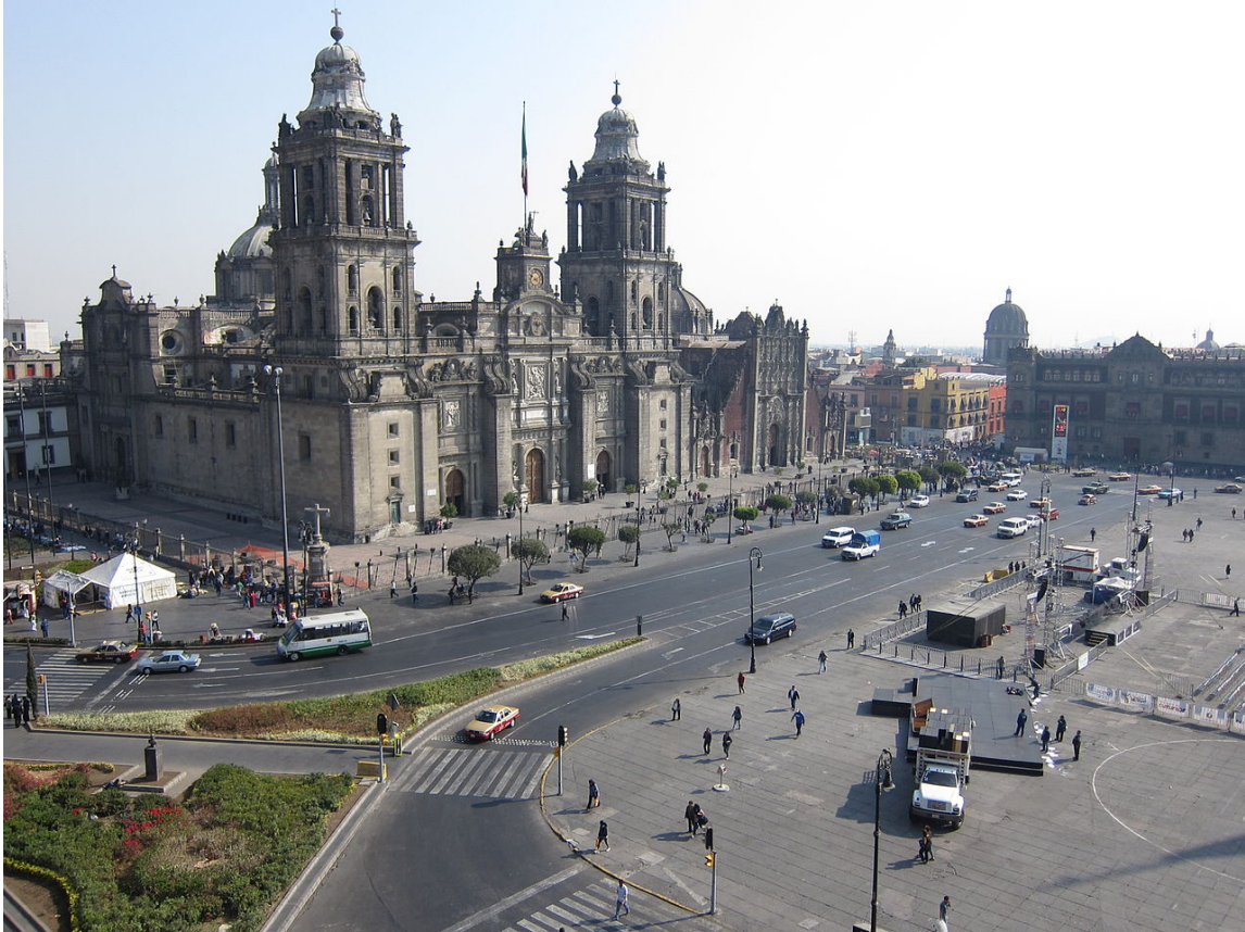
Figure 5.13: Mexico City Metropolitan Cathedral, Mexico (Courtesy of Jeff Kramer, Wikimedia Commons)
